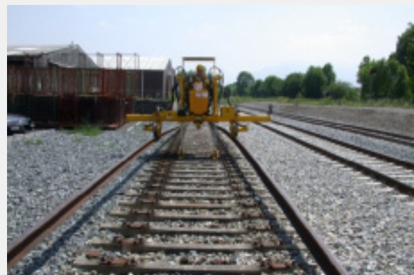
Continuous, steady placement of rails on the sleepers at the requirement gauge with ROTHREAD
