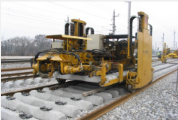
Temporary storage of the sleepers on track then transport and lay Sleeper in track with second unit
